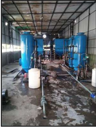
Sewage Treatment Plant
